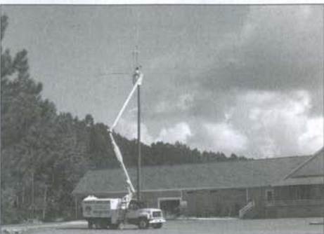
N7BHC/B - installation of the 17 ele beacon yagi
